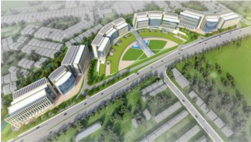
Figure 7: The World Trade Center in New Delhi, India with IP500 infrastructure and IoT OEM applications
